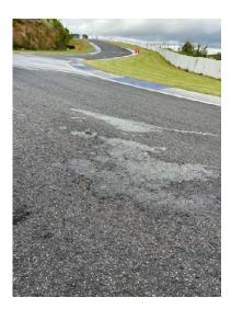
This photo shows water seepage through the track just prior to the finish line. There is a significant bump on the track, even though this is probably not noticeable in this photo. We are lucky that the seepage is not actually on the racing line.
